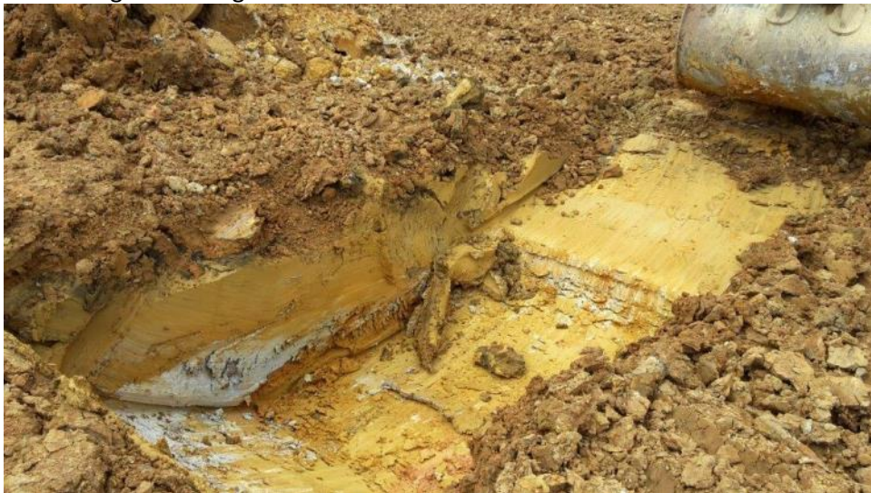
TP1 through the soft ground
