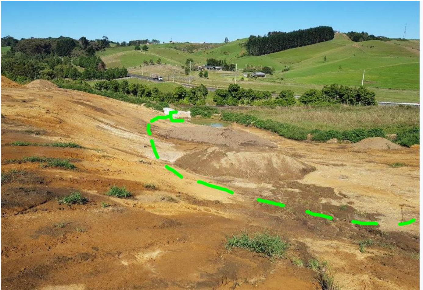
Requested underfill drain in green.
