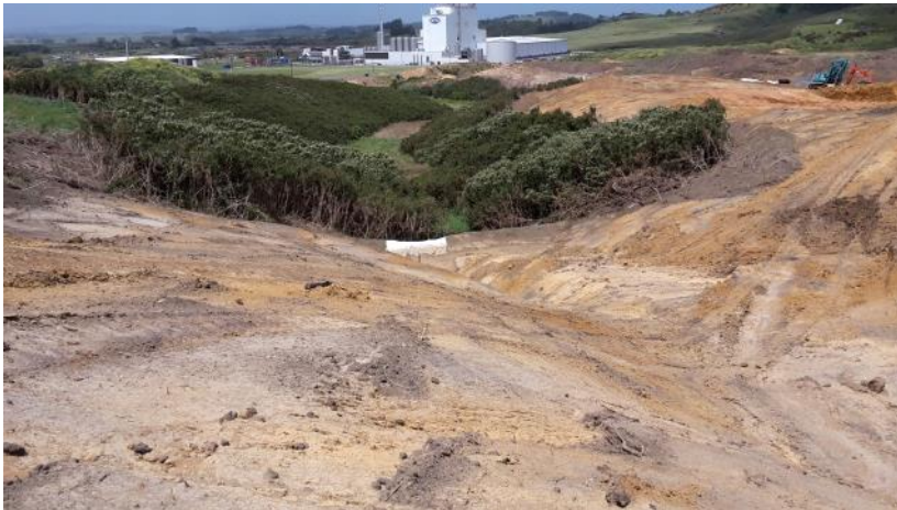
Fill N gully mucked out
