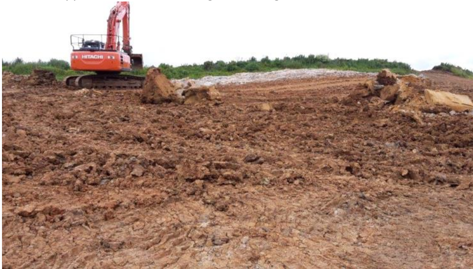
Area of soft ground
