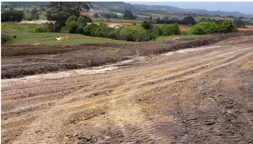
Haul road stripped
