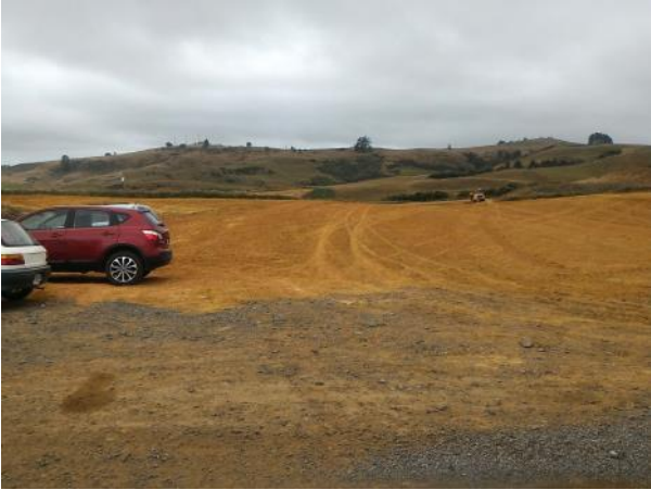
Fill M to Cut 10
