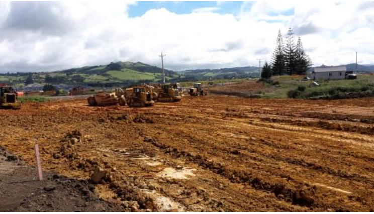
Fill M looking to road
