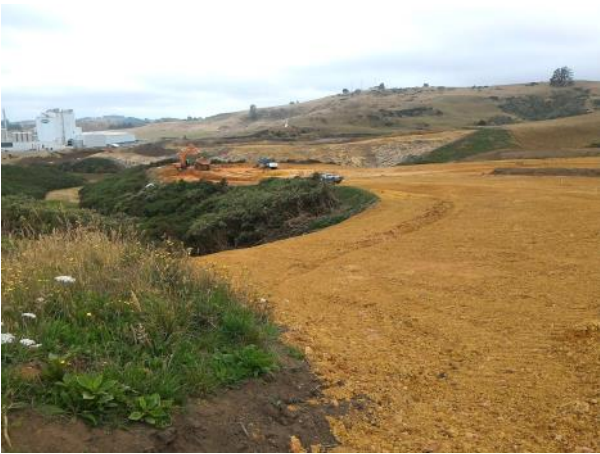
Toploading at cut 10, almost completed
