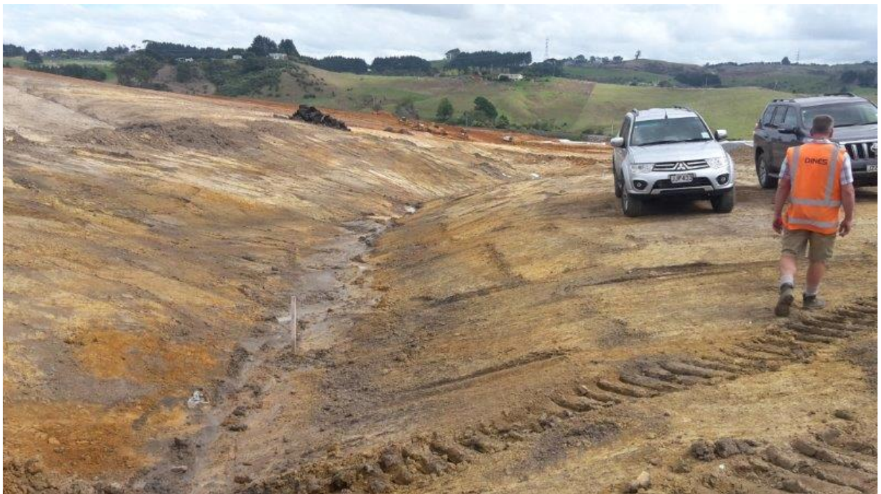
Top of gully - needs drain run up as chimney drain once fill cover less than 2m to tap spring and ensure adequate coverage over drain is maintained
