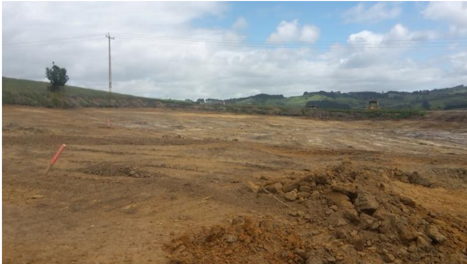
Fill M topsoil strip
