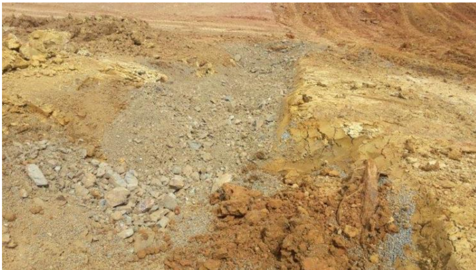
Spring area at base of gully (near subgrade level). This area is under road and just needs to be treated as necessary to build road.
