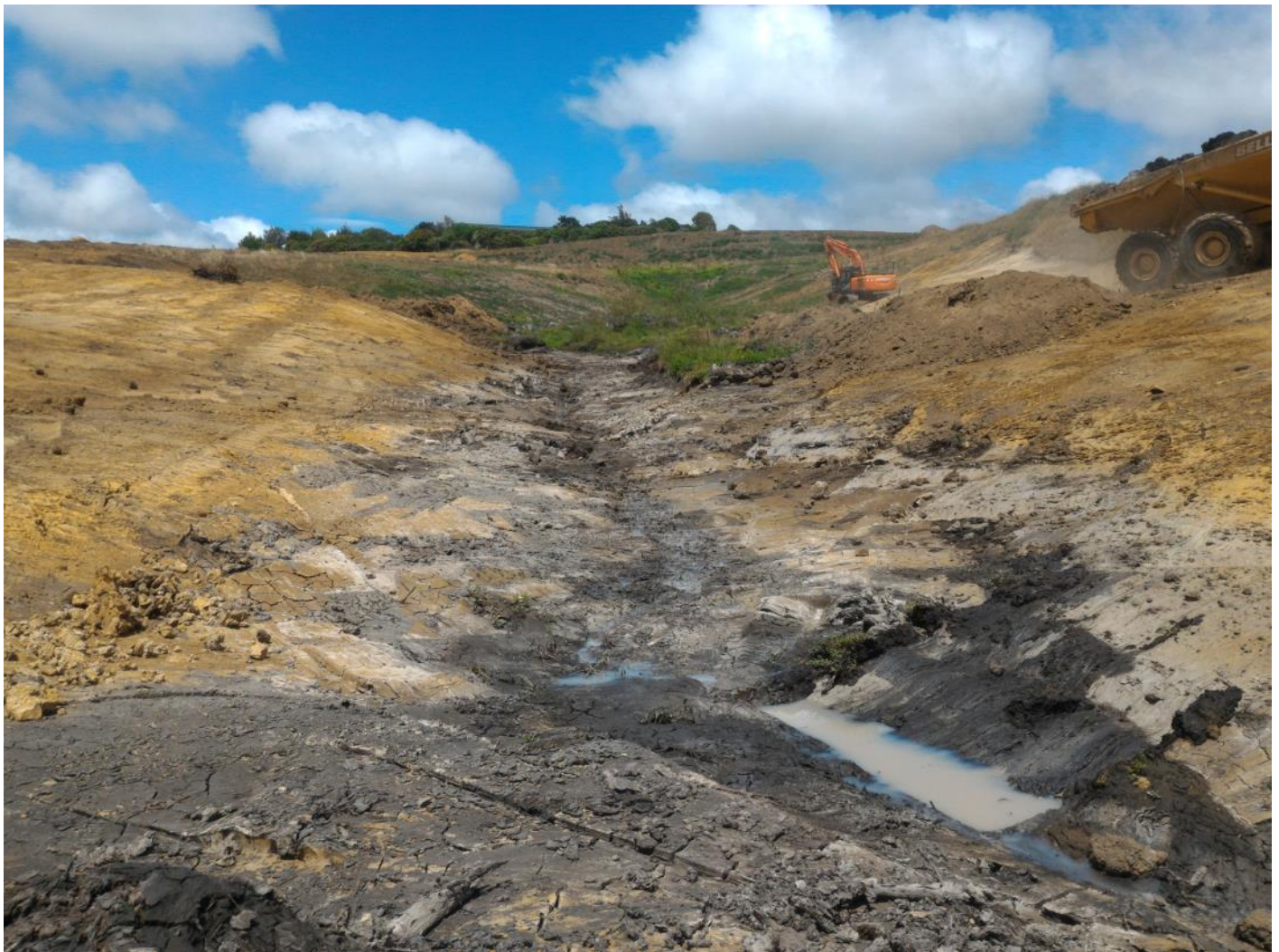
Looking upslope at fill I
