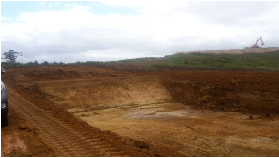
Silt pond 8 preparation
