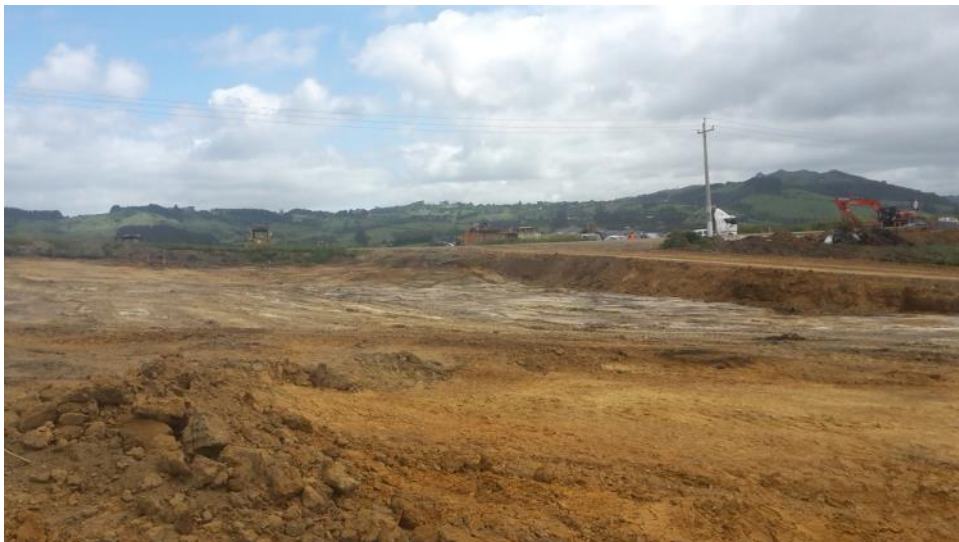
Fill M topsoil strip
