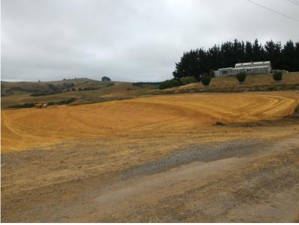
Fill M to Cut 10
