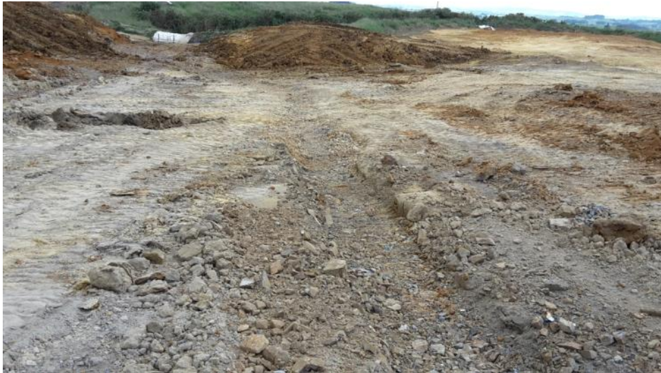
Fill M subsoils
