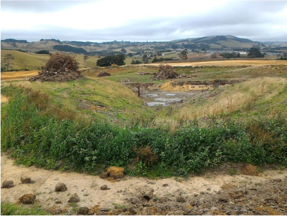
Fill P tributary gully
