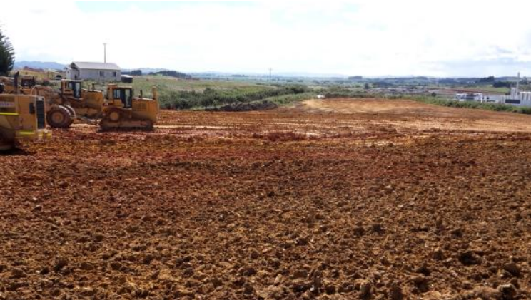
Fill M looking east downslope to gully
