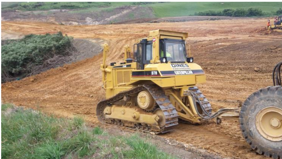
Fill N materials being dropped
