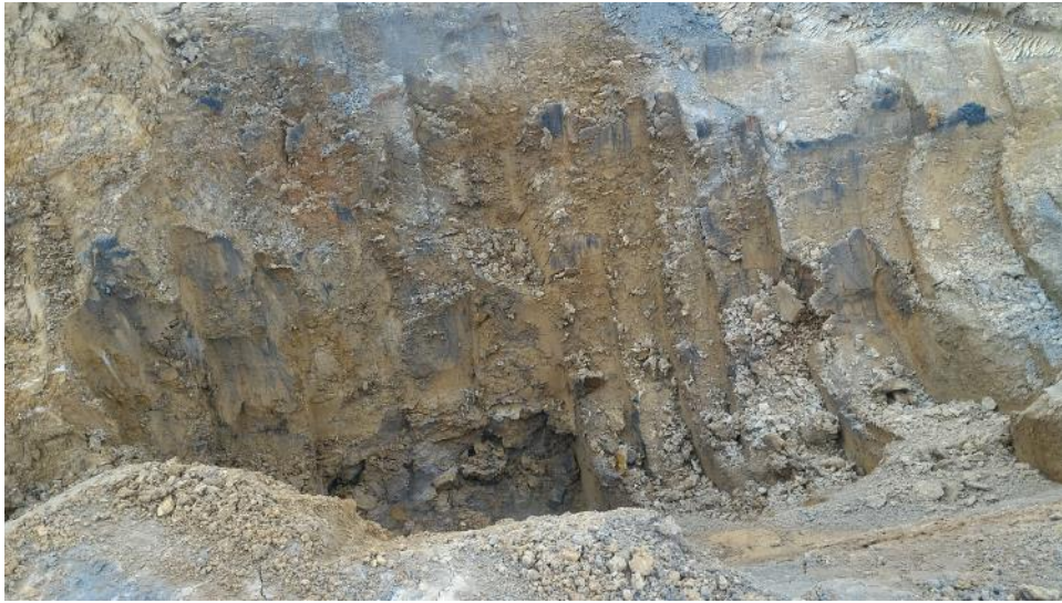
4m deep pit at contaminated area undercut
