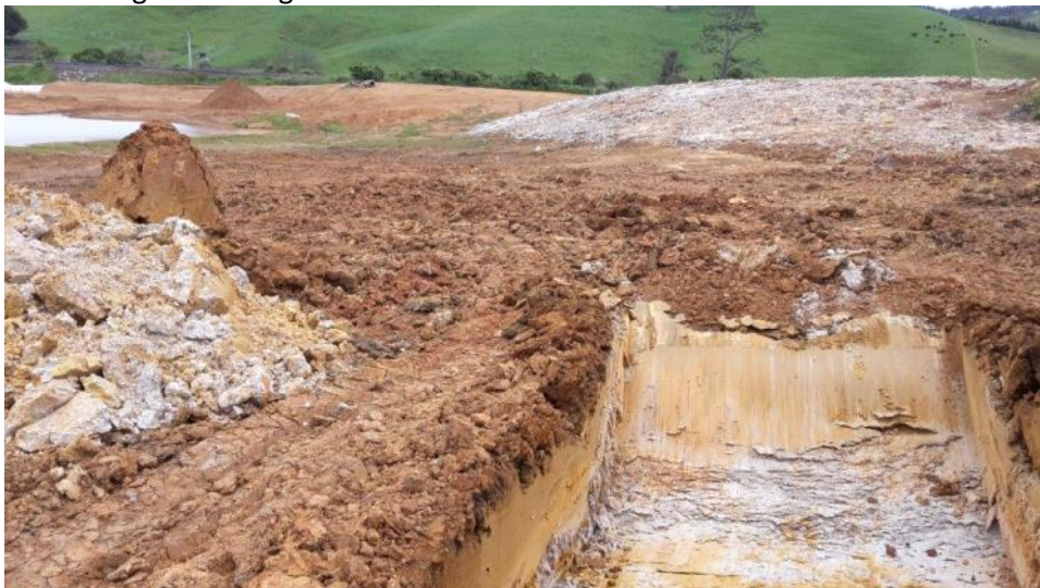
TP2 through the soft ground
