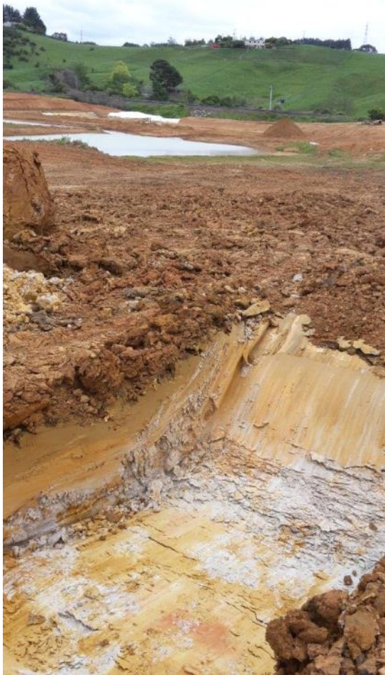
TP1 through the soft ground
