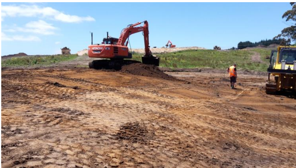
Pond 8 topsoil stockpile being moved
