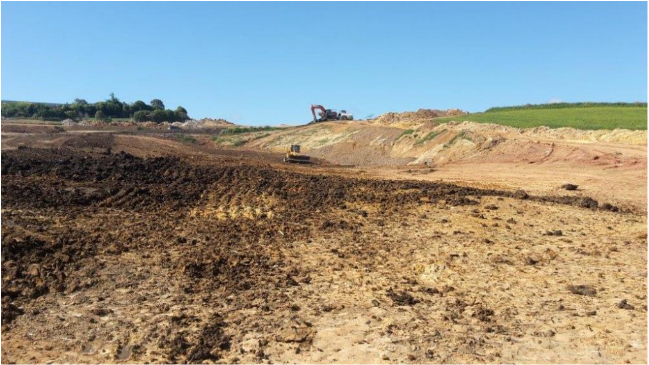
Fill 1 - SPR blanket located near where compactor is.
