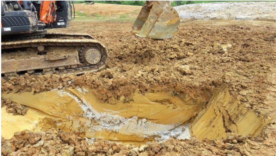
TP1 through the soft ground
