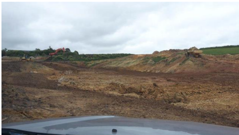
Fill 1 - there is an area of seeping groundwater on the right face of the gully- Trevor is going to extend the SPR blanket up this face and tap into the underfill drain in the area.
