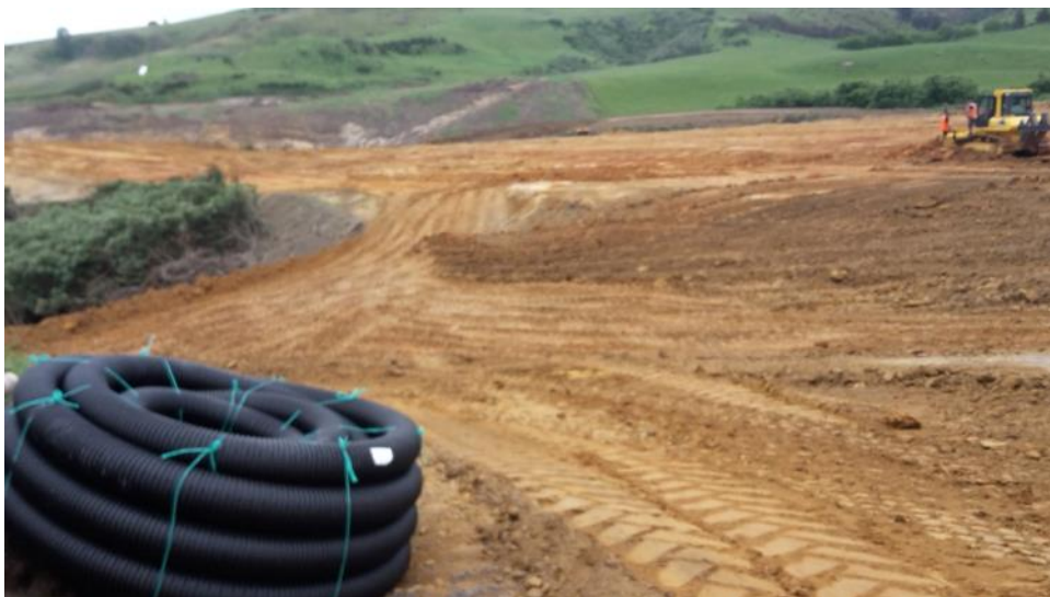
Fill N gully being filled
