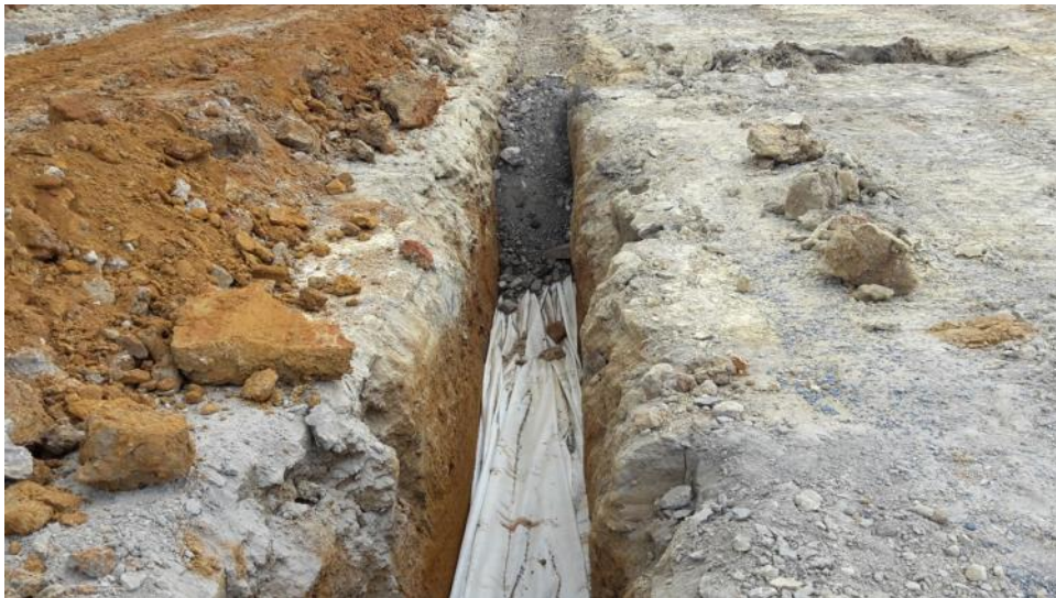
Fill M subsoils
