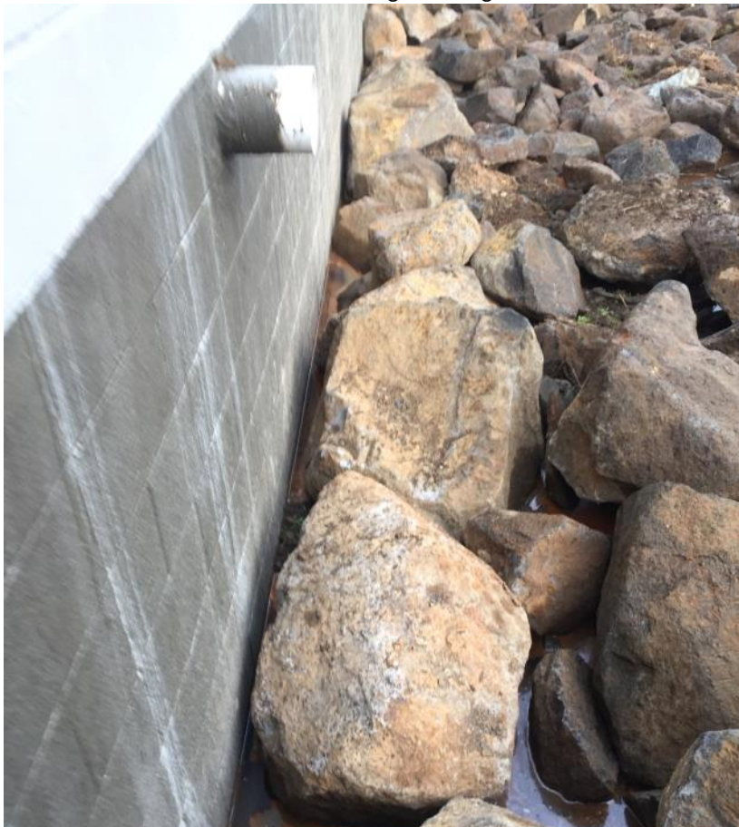
Outlet for the other underfill drain through the stage 3B Pond weir
