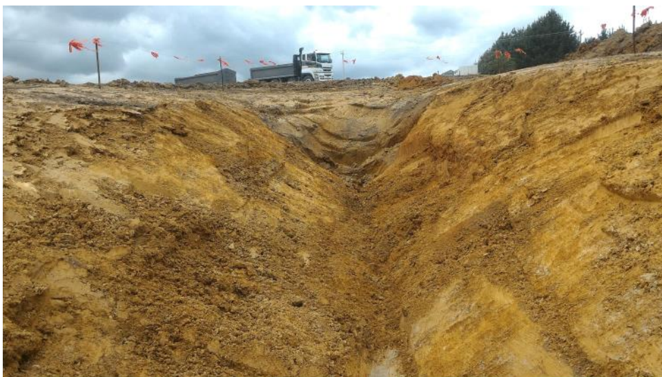
Looking up contaminated area undercut
