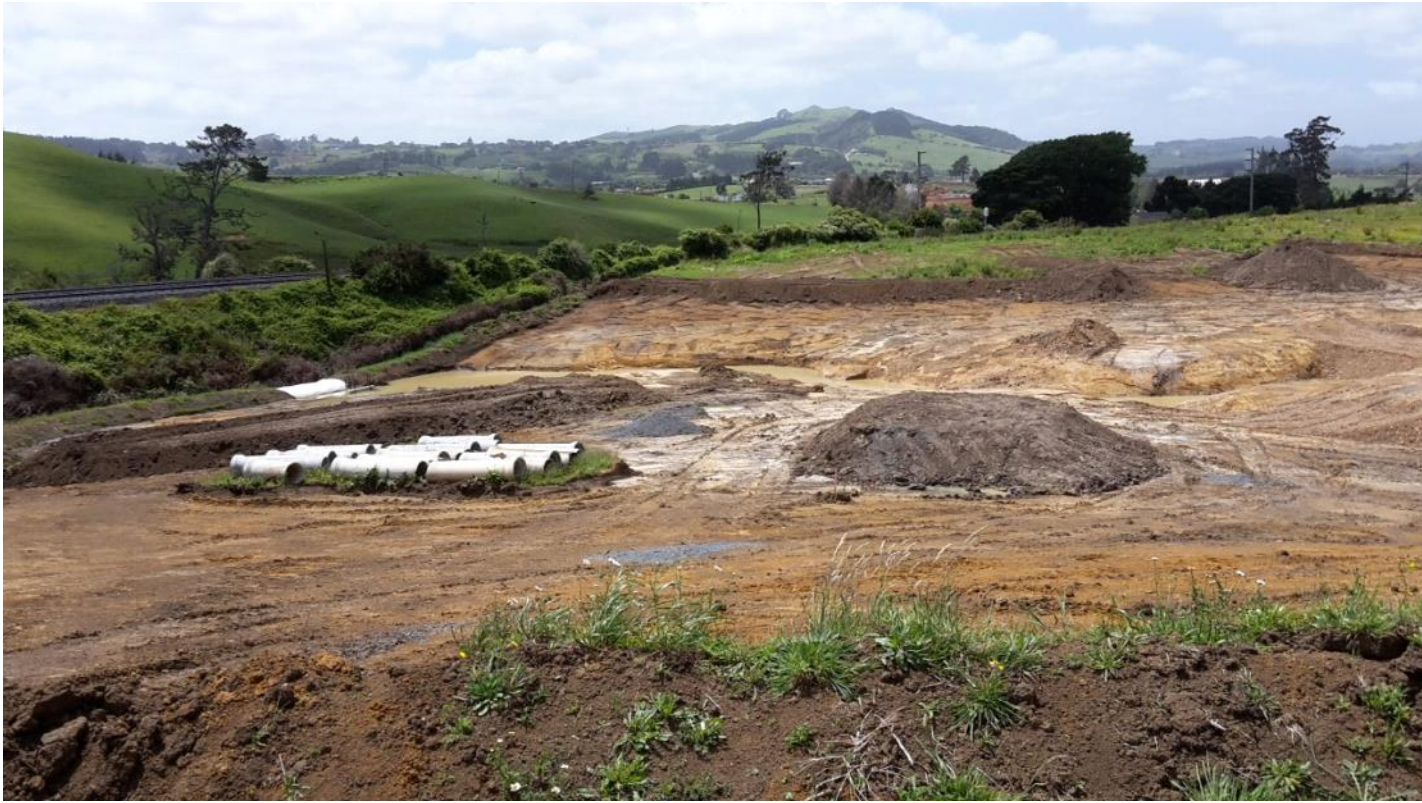
Pond 8 stripped with topsoil needing removal
