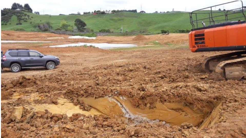
TP1 through the soft ground
