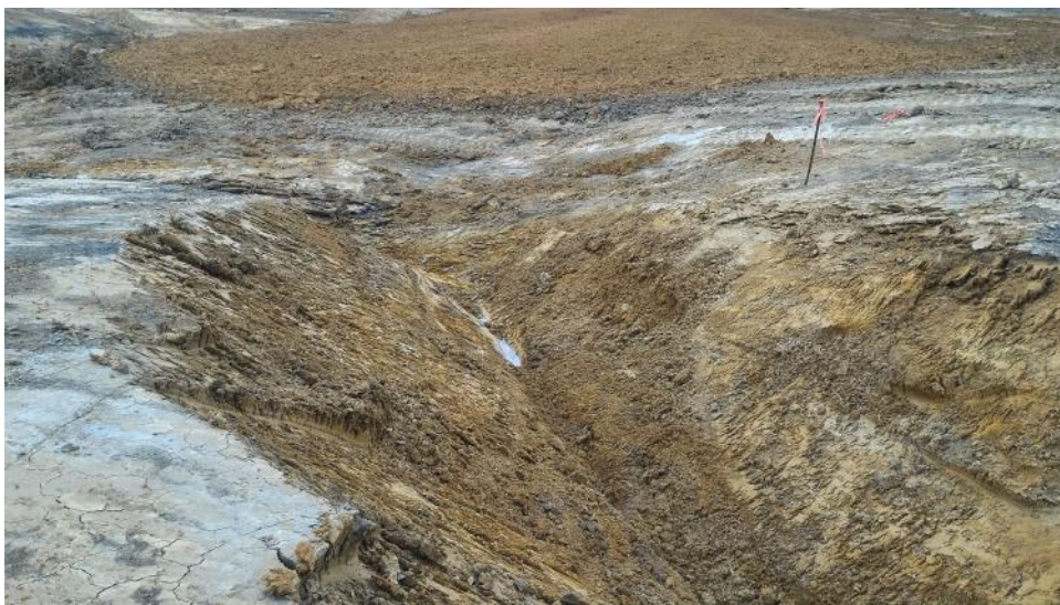
4m deep pit at contaminated area undercut
